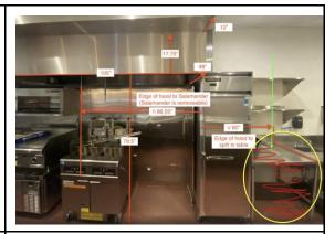
The salamander on the left needs to be removed or moved to the left closer to the edge of the left-hand side of the hood.
