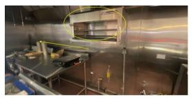
The shelving on the right-hand side of the wall above the SS table needs to be removed or placed more on the right above the sink area.
